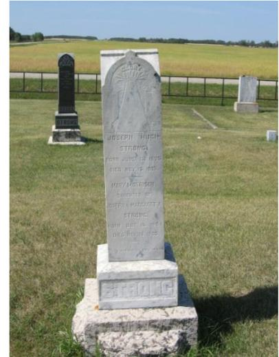
Some bases, whether slot-type or flat-top, usually protrude above grade from about two inches up to the full height of the base. Cast concrete bases are usually set slightly below grade (i.e., not visible).
